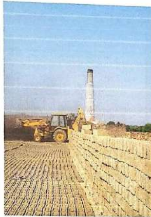
Brick making by clay at LBFA Brickfield
